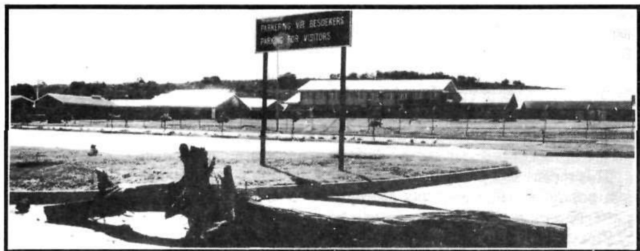
The unopened Lenasia Hospital: Parking place but no one to visit
